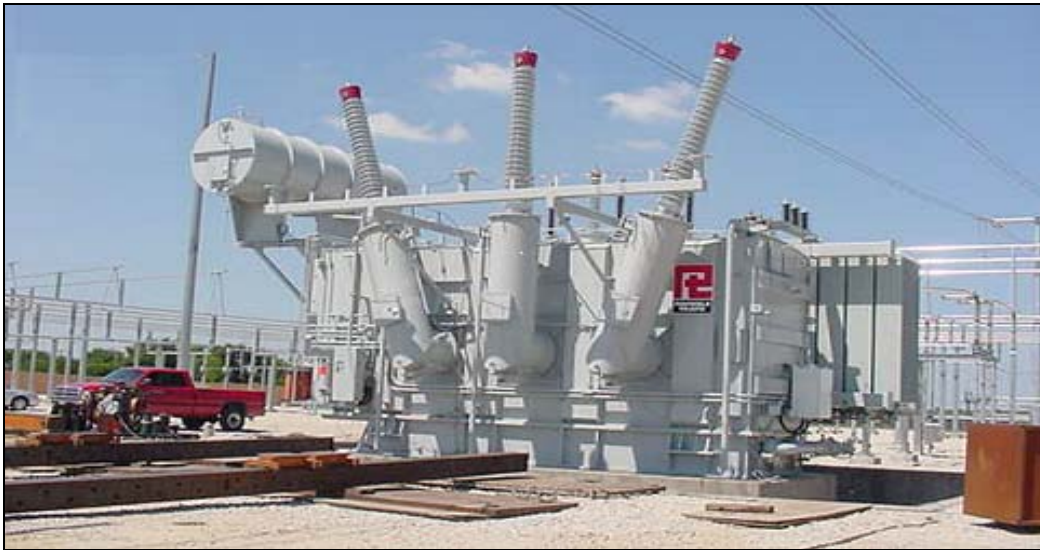
Figure 5. 345 kV Transformer Installation
