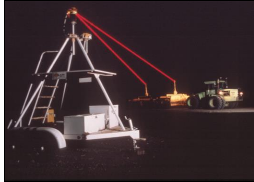
Figure 11. Laser-Leveling Irrigation Land
