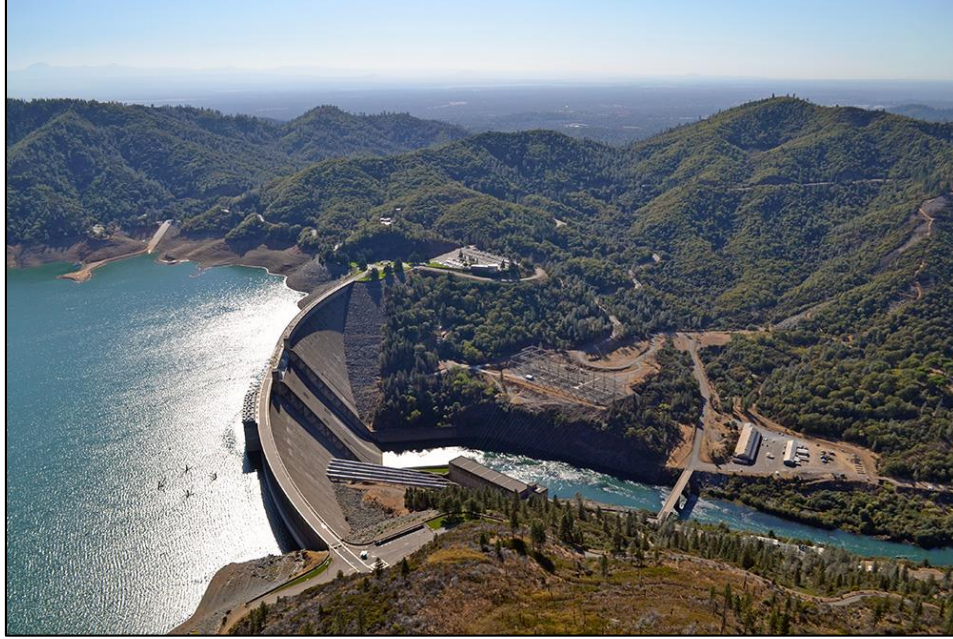
Figure 2. Shasta Dam and Reservoir
